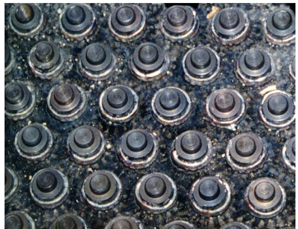
Studs are installed in a matrix pattern
